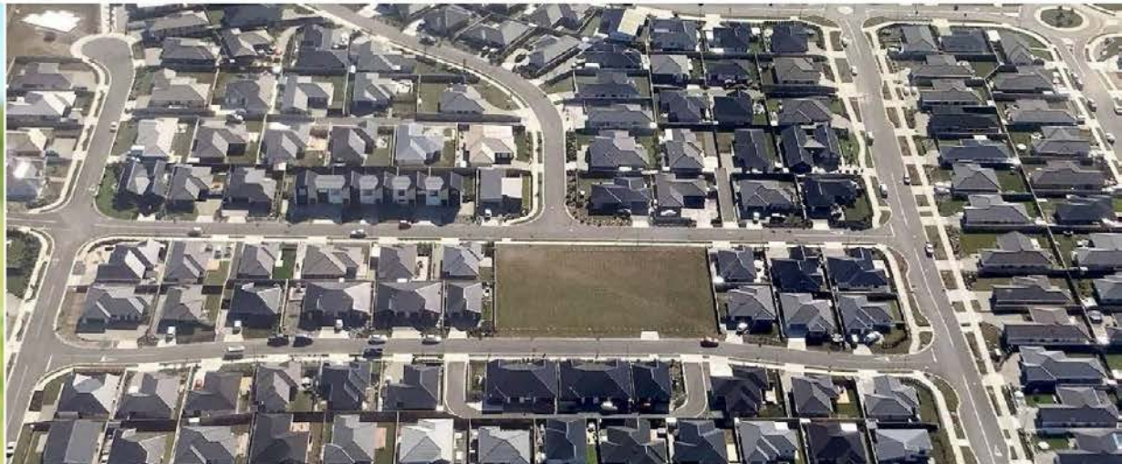
Berryfields subdivision in Richmond / greenfield development
